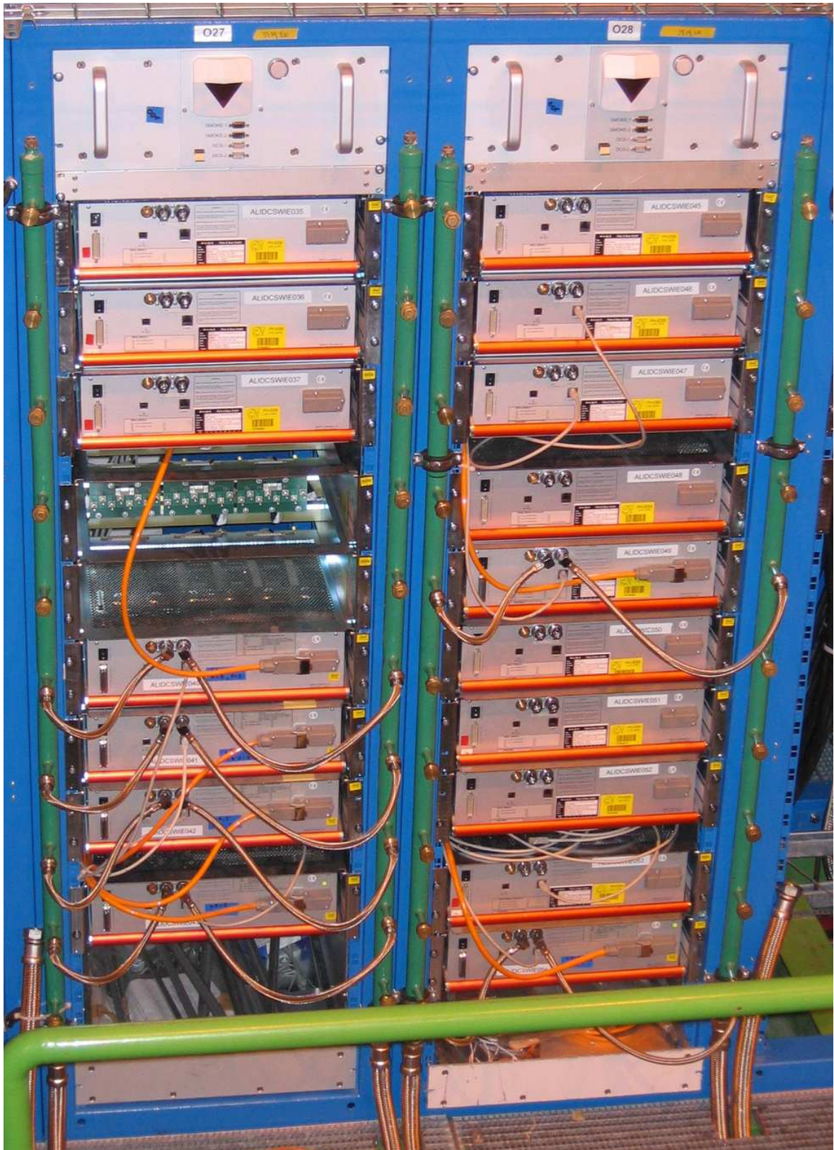
Figure 4.1: Photo of two racks with low voltage supplies during installation. Once fully equipped these two racks will power 4 super modules.
