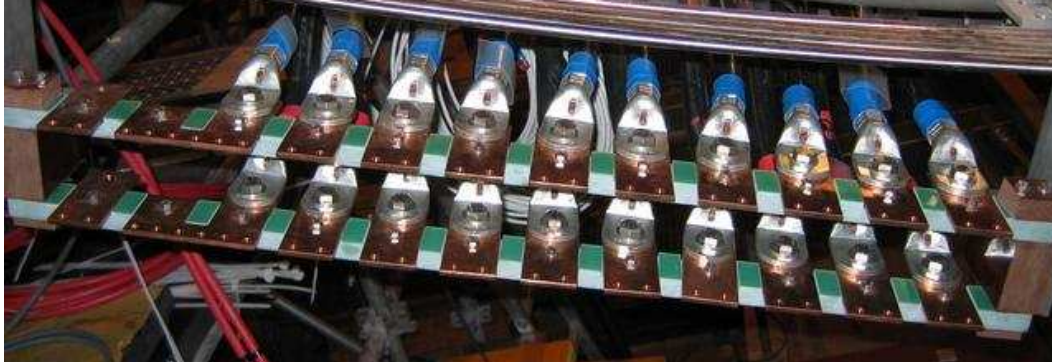
Figure 4.2: A low voltage patch panel, here sector 14 in the baby frame.
